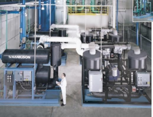
Three 9000 scfm (255m<sup>3</sup>/min) Hankison HEDS Series Drying Systems furnish clean, dry air to a major automobile assembly plant. Two component system allows use of existing space.
